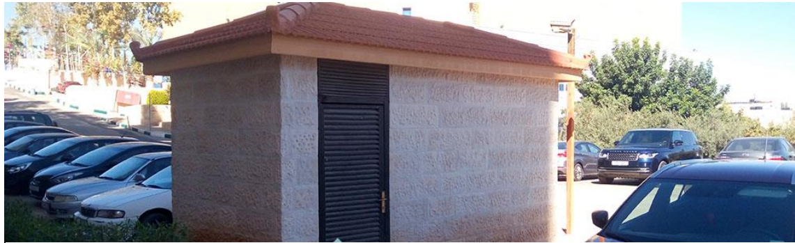
Water Saving Well (This room includes the water compressors)
